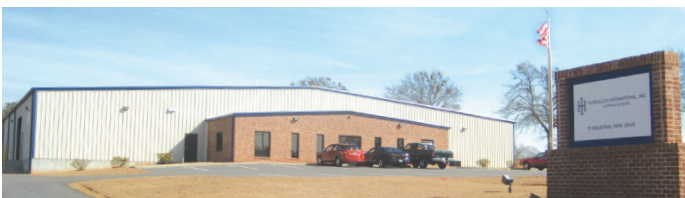
AIRCRAFT COMPONENTS AND GSE MRO FACILITY
